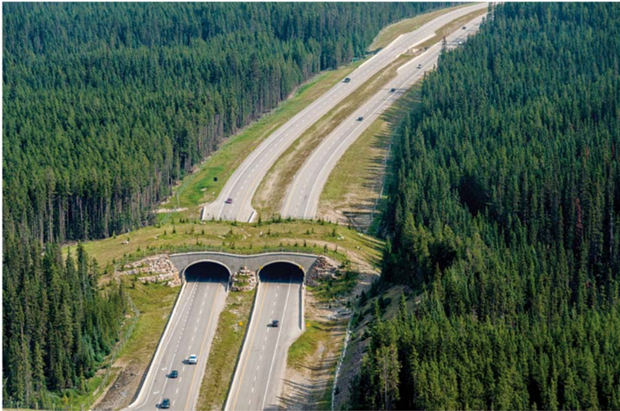
Aerial image of wildlife overpass on the Trans-Canada Highway (#1) in Banff National Park (Image courtesy of Parks Canada)
