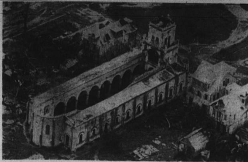
DEVASTATION — Most of the Catholic churches in Haiti were devastated by Hurricane Flora. This is an air photo of the church at Aquin where many Haitians who sought refuge from the storm were killed when the roof collapsed.
