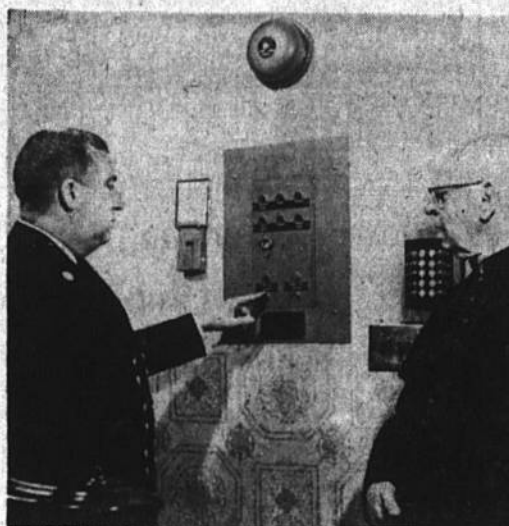
FIRE INSURANCE — Westfield Fire Chief Martin D. Burke reviews the operation of the control panel for an elaborate fire detection system installed by the Walter Kidde Co. at Holy Trinity, Westfield, with Msgr. Henry J. Waterson, pastor. The system pinpoints the exact location of any fire and is connected with the Westfield fire station.
